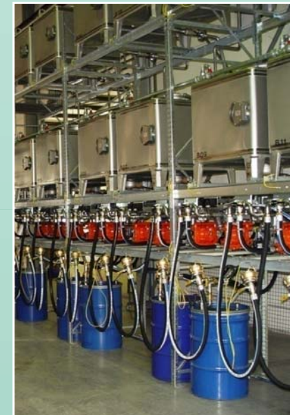
Combination of stationary tanks and 200 l-barrels for printing inks and additives
