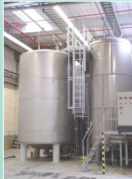
20 m 3 - and 30 m 3 -tanks for the storage of resins
